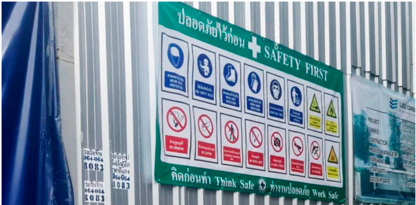
Image 1 Safety instruction in a Construction Site at Ekamai
